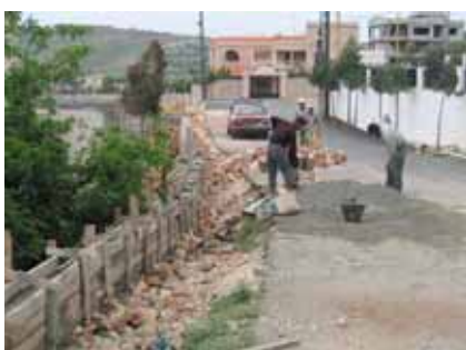
Working on support walls
